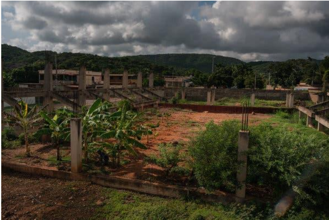
A worker plants bananas and plantains on an old half-built stadium outside the Augusto D'Aubeterre Bolivarian school.
